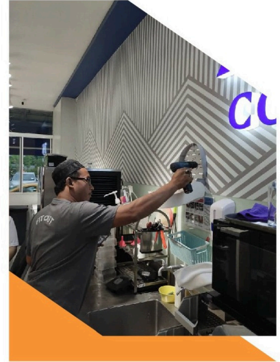
FINISHING & PAINTING WORK
