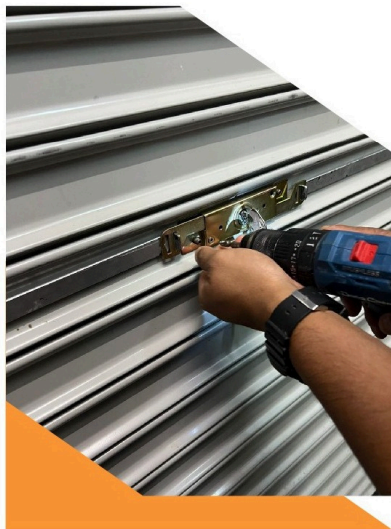
DOOR, WINDOW & ROLLER SHUTTER WORK
